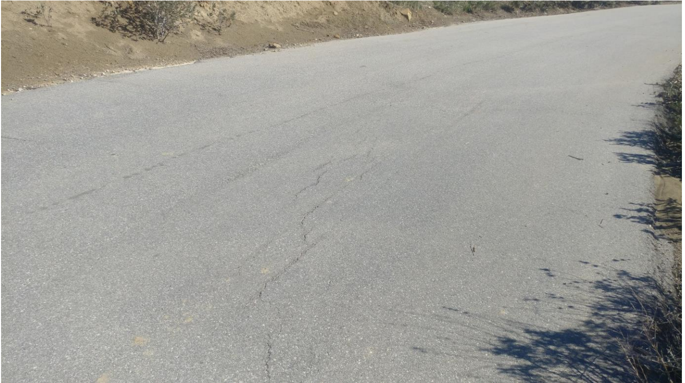
Photo 3 – Cracking at Lower Site (S2)
