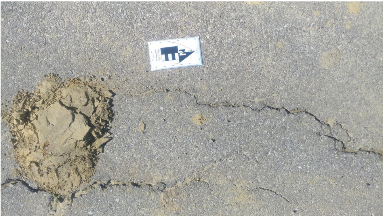
Photo 2 – En-Echelon Fracturing at Site 1
