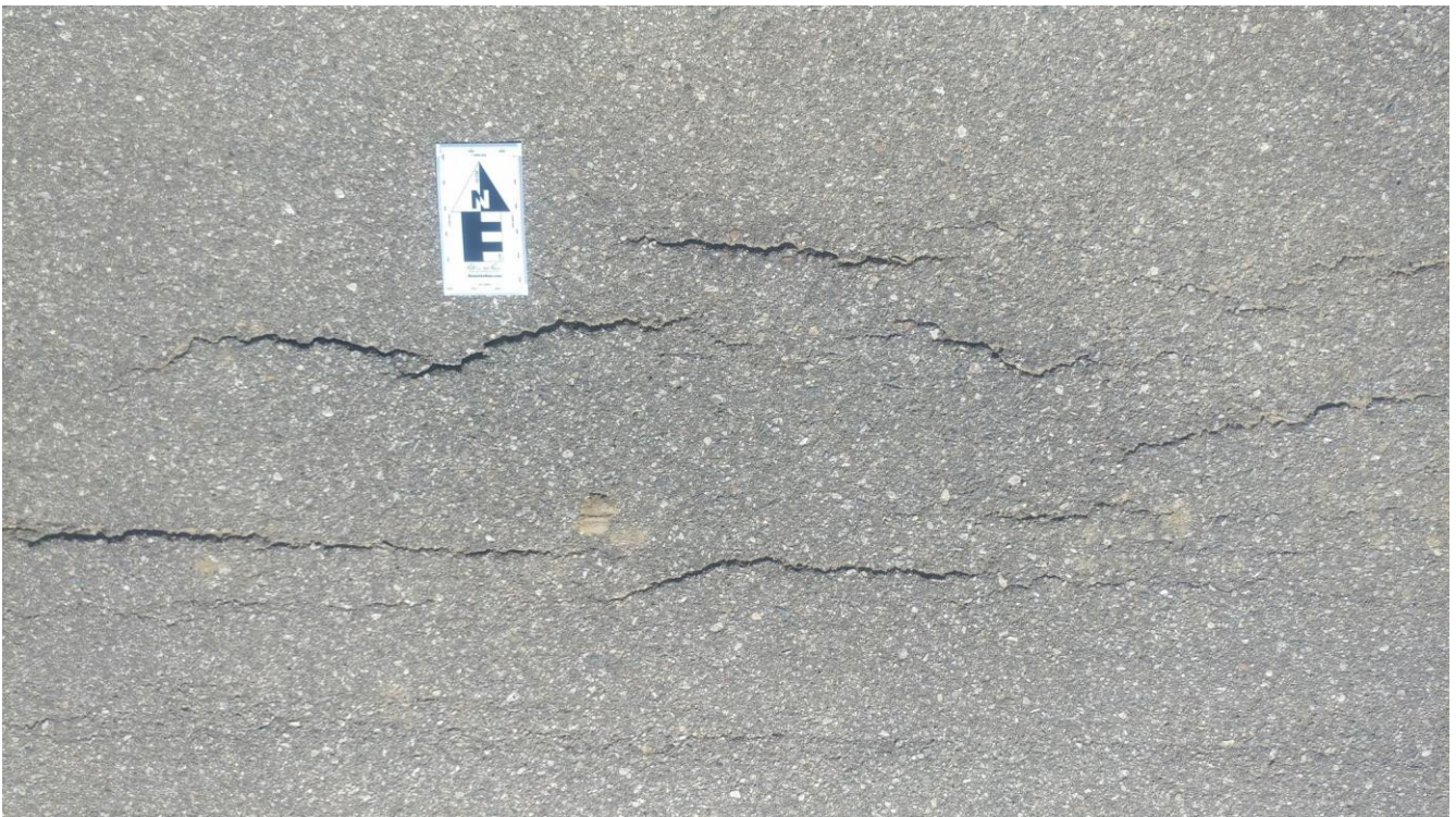
Photo 4 – Area of uplift and fracturing
